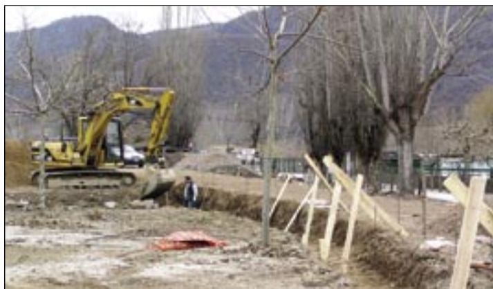
Baustelle Kalterer See
